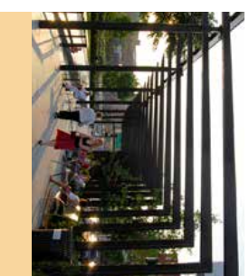
Fig. 7.3.127 Bespoke Shelter: Powdercoated Aluminium
