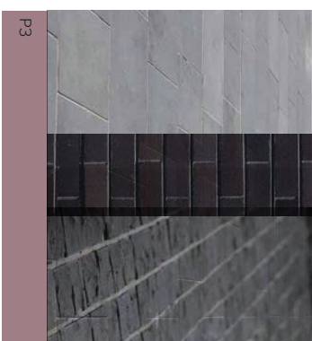
Fig. 7.3.113 COS Concrete Unit Paver with Concrete Setts, with Hamlet Blue Brick Banding
