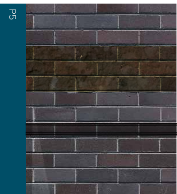
Fig. 7.3.115 Hamlet Blue Brick with sandstone inlay and metal inlay
